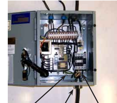
Motor Ground Lug Cord Grip Motor Wires 2T1, 4T2 Motor Ground
