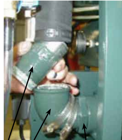
Pump Exhaust Pipe Pump Exhaust Elbow Pump Exhaust Elbow Locknut
